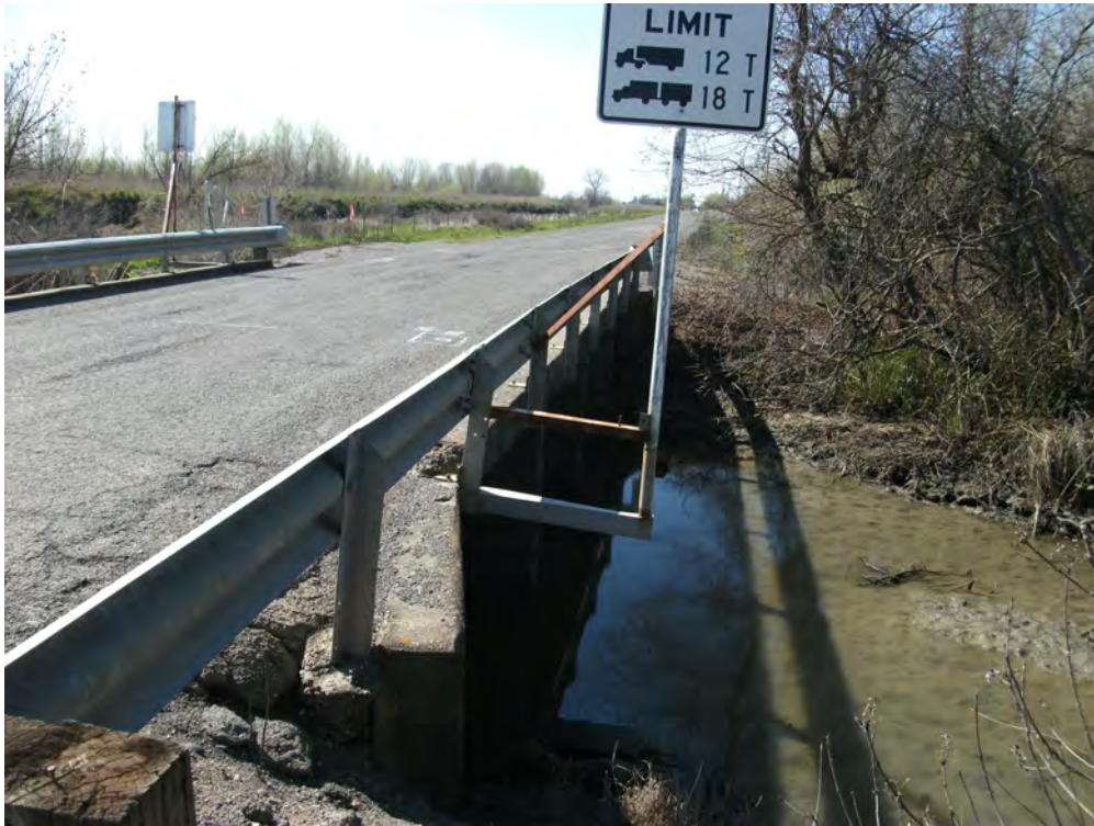
9. Looking West along North Side of Bridge No. 11C-0179
