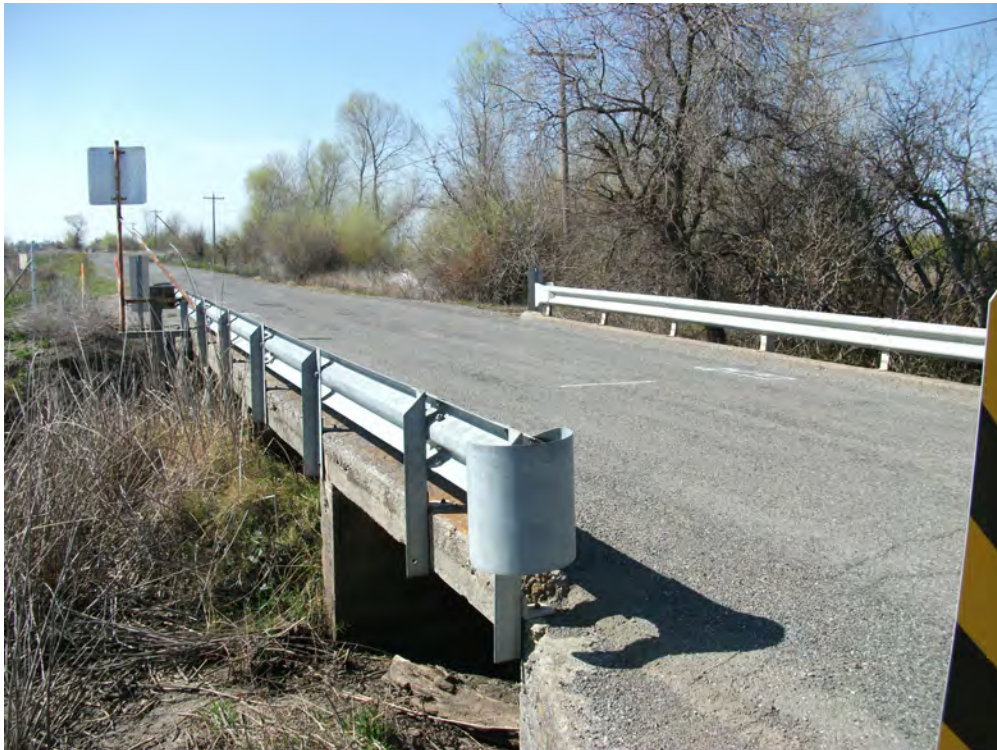
8. Looking West along South Side of Bridge No. 11C-0179
