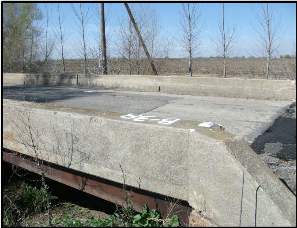
2. Southeast Corner of Bridge No. 11C-0015
