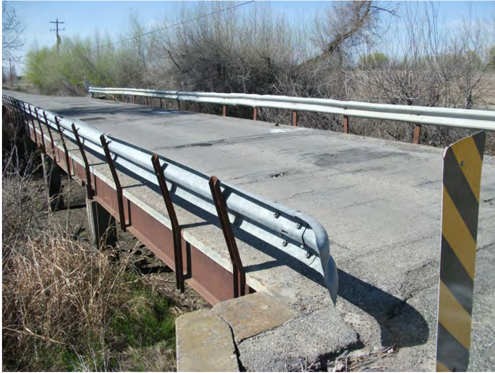
7. Looking West from Southeast Corner of Bridge No. 11C-0016
