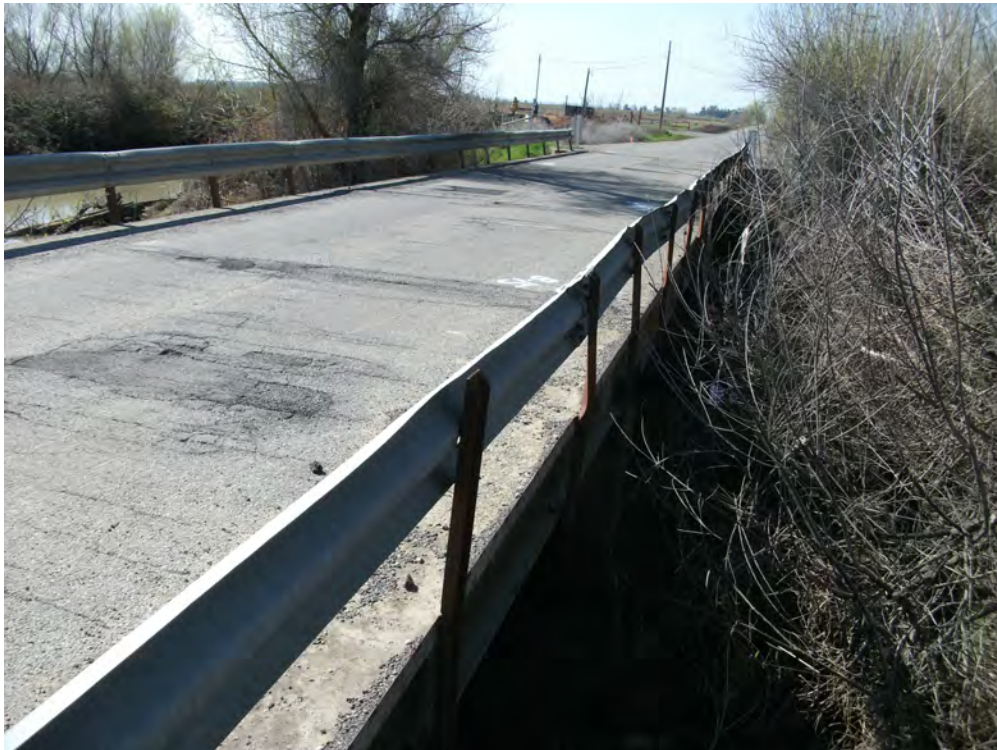
6. Looking West along North Side of Bridge No. 11C-0017
