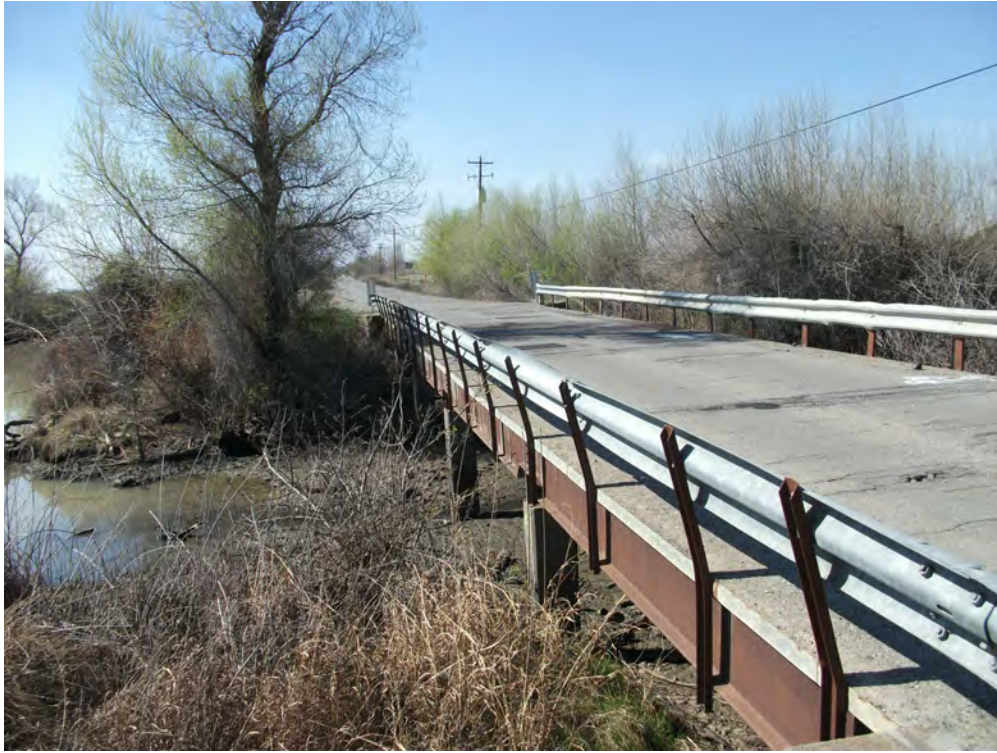
5. Looking West along South Side of Bridge No. 11C-0017
