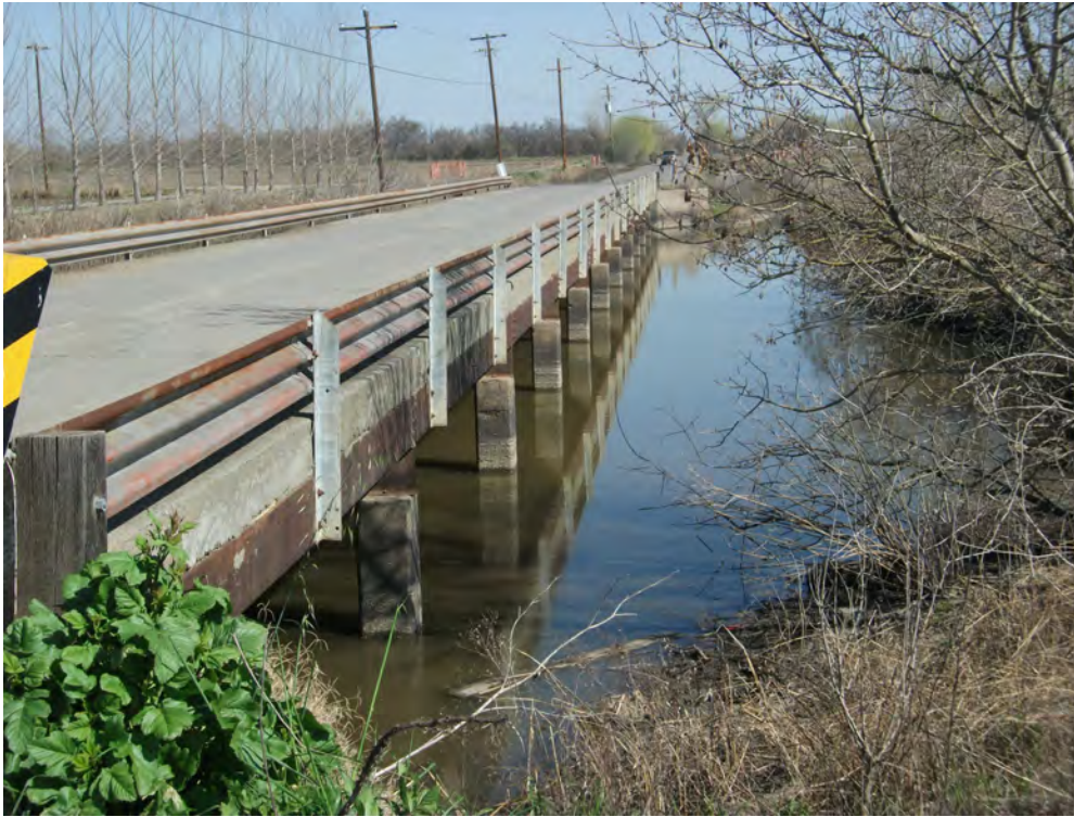
3. Looking East along South Side of Bridge No. 11C-0016
