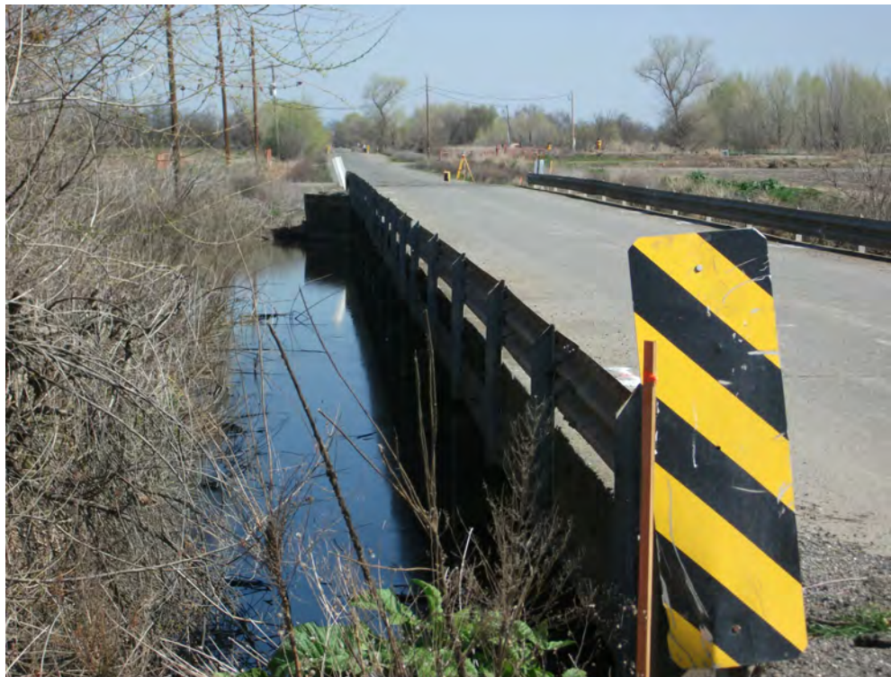
4. Looking East along North Side of Bridge No. 11C-0016
