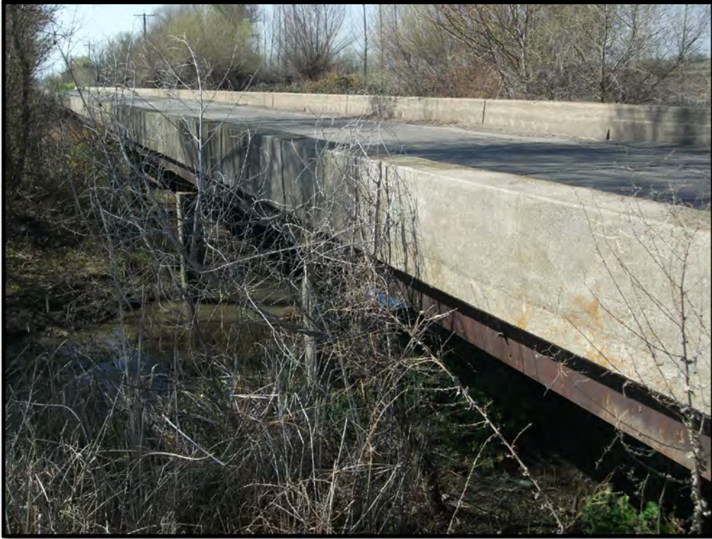
1. Looking West along South Side of Bridge No. 11C-0015
