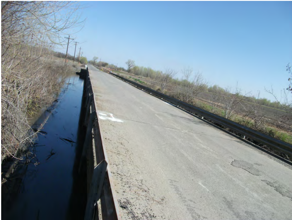
10. Looking East along North Side of Bridge No. 11C-0179
