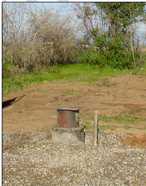
Photo 1. Test Production Well Prior to Pump Installation.
