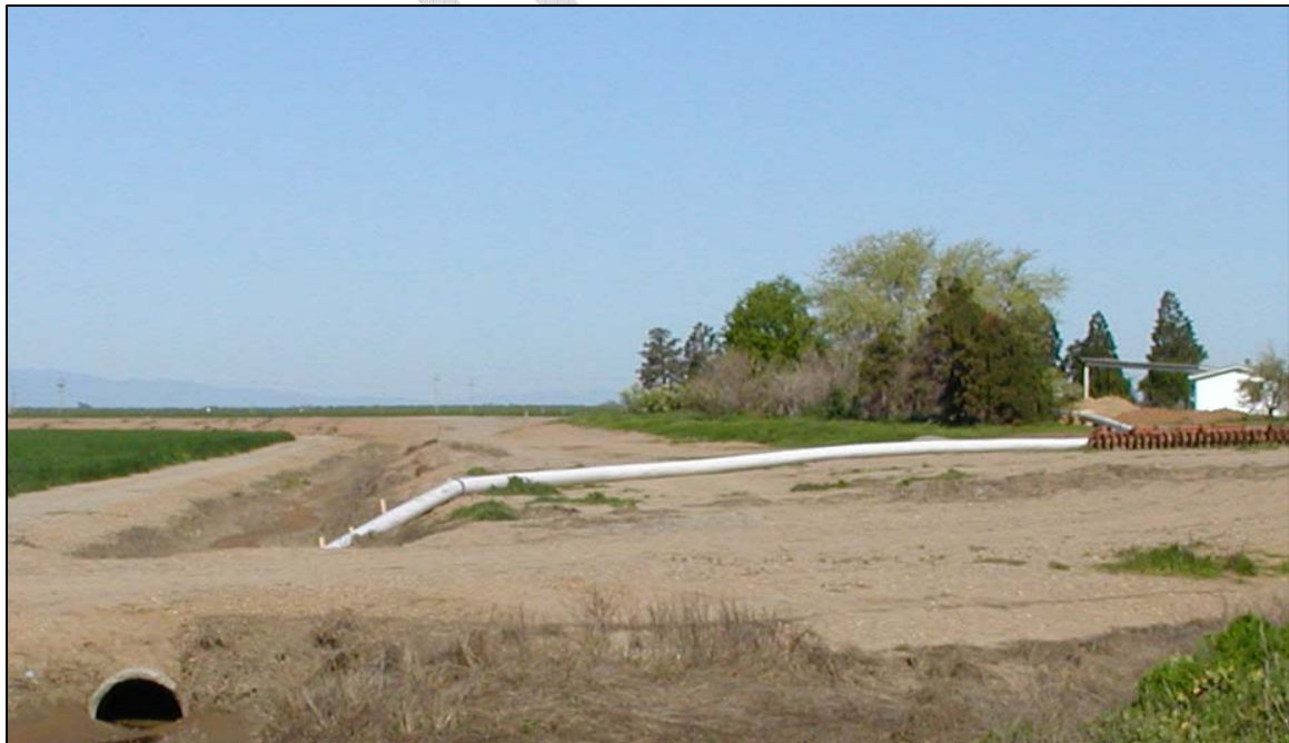
Photo 2. Conveyance Pipe to Existing Drainage System.
