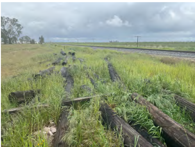
View of wooden railroad ties.
