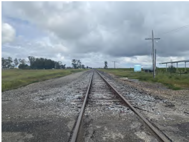
View of railroad easement and spur, facing north.
